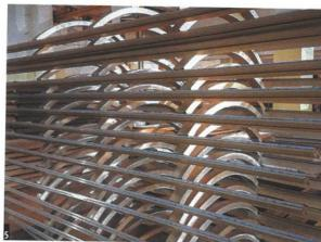
ventilated systems also create active air movement behind the cladding – thus preventing hot air build-up between the cladding and the wall." The benefit of this kind of cladding is that it reduces indoor air temperature by a few degrees.
